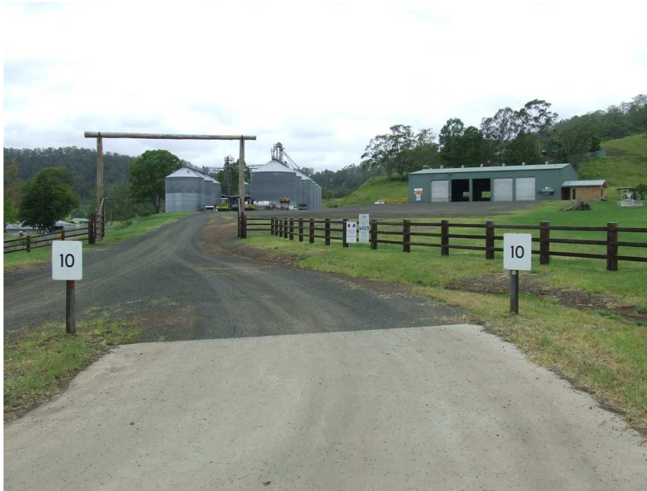
Figure 2 Site viewed from Kyogle Road entrance
